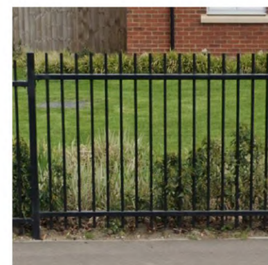
Black metal railings to replace removed brickwork panels in front boundary wall - See street scene drawing for locations
